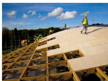
FIGURA 6: RECOBRIMENTS FLEXIBLES. PVC A MANNHEIM I Tauler CONTRALAMINAT A SAVILL GARDENS. ©: WWW.FOURTHDOOR.ORG
