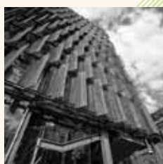
CH2 Building City Council. Mark Pierce Design, Inc. SOSTENIBILITAT.
