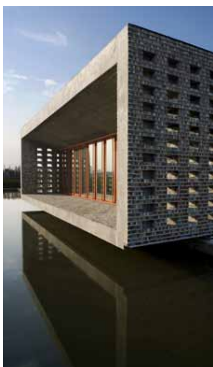
CERAMIC HOUSE, 2003-2006, A JINHUA. FOTO: LV HENGZHONG
