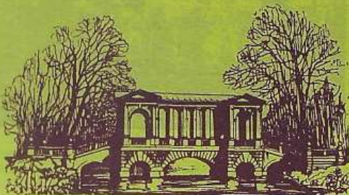
Palladian Bridge, Wilton.
